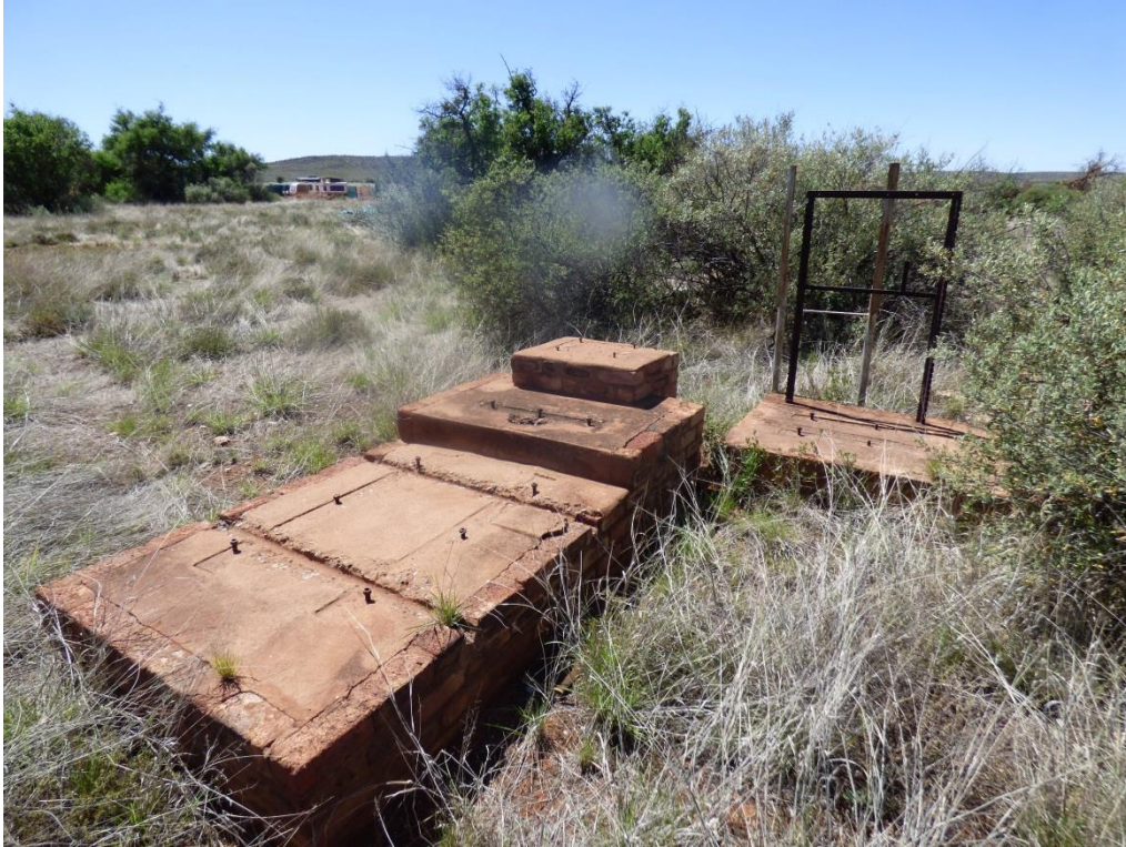
Figure 16: Brick and cement platform, which might have housed a generator or pump relating to borehole irrigation. Younger than 60 years of age and outside of the western footprint boundary (courtesy Ubique).
