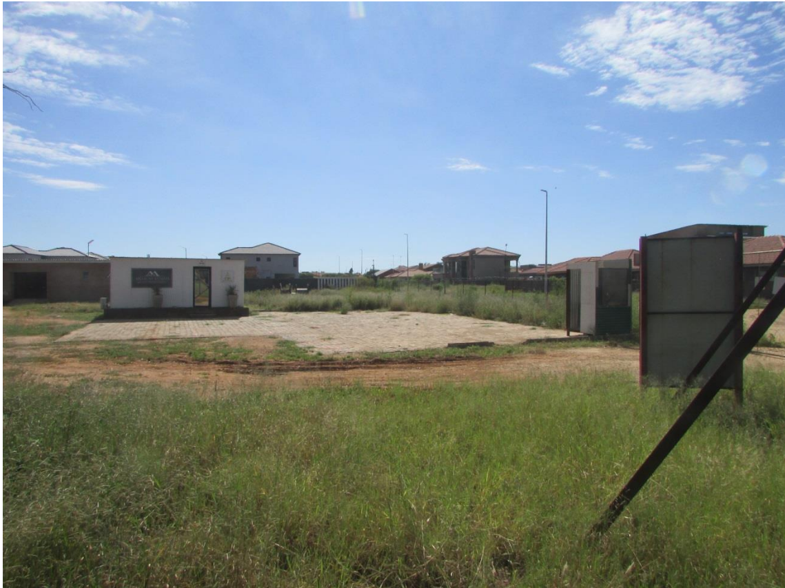
Figure 11: A view of the area with the Site Office visible. Taken towards the east with the southern boundary visible.
