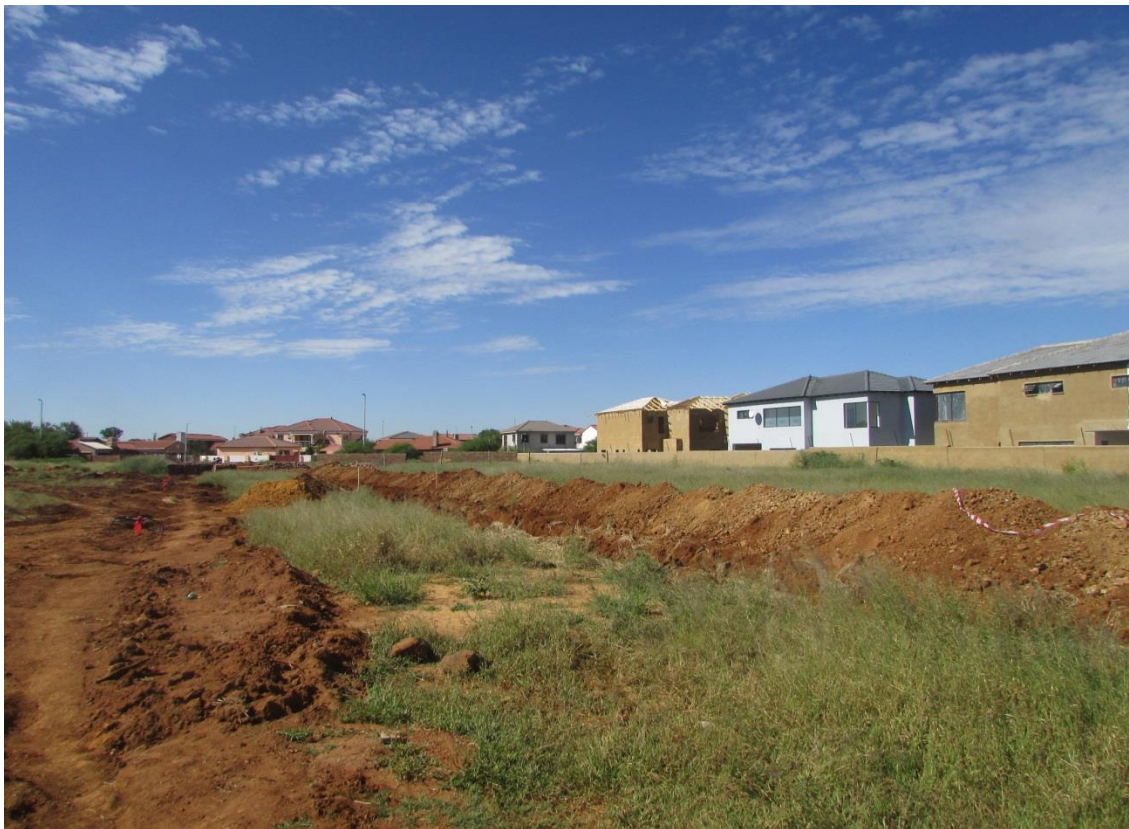
Figure 4: Another view of a section of the development area. Note the already existing housing and trench for services.
