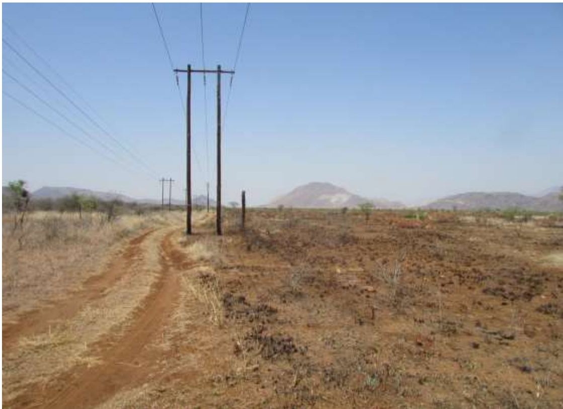
Figure 7: Powerlines and servitudes have also impacted on the area.
