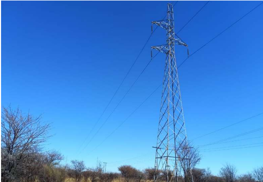
Figure 3: Eskom Powerlines has impacted on the area (courtesy Reach Archaeology).
