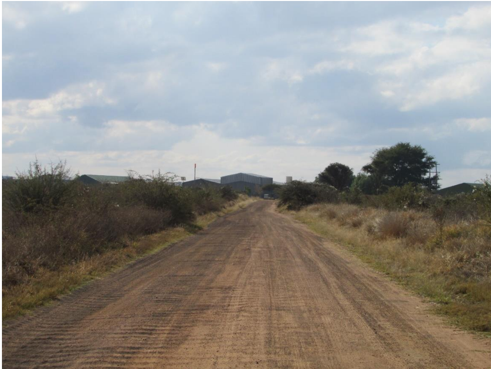
Figure 10: The road towards the existing Airfield with the associated infrastructure there.
