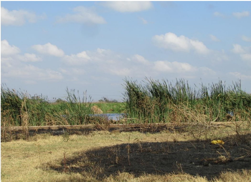
Figure 13: A view of the existing sewer ponds (Waste Water Treatment Works).
