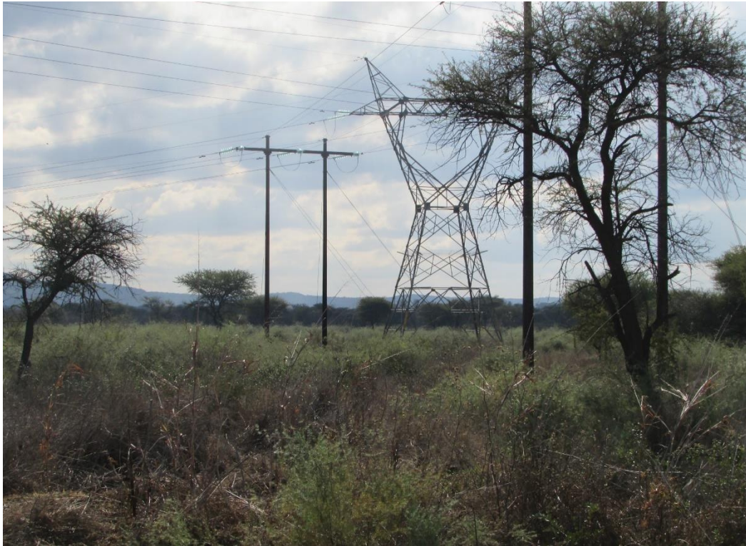
Figure 8: A view of a section of the study and development area. Note the fairly dense vegetation, as well as the Eskom Powerlines and servitudes.
