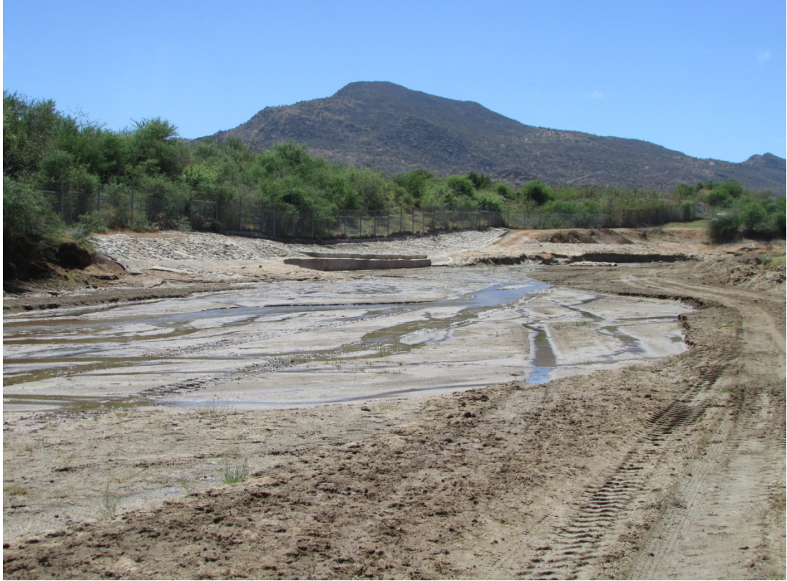
Figure 5: Another section of the Point 1 rehabilitation area.
