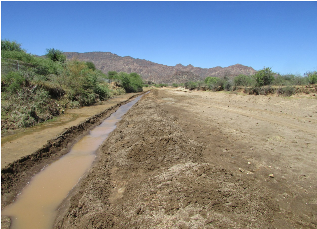
Figure 6: Another view of the work being done at Point 1.
