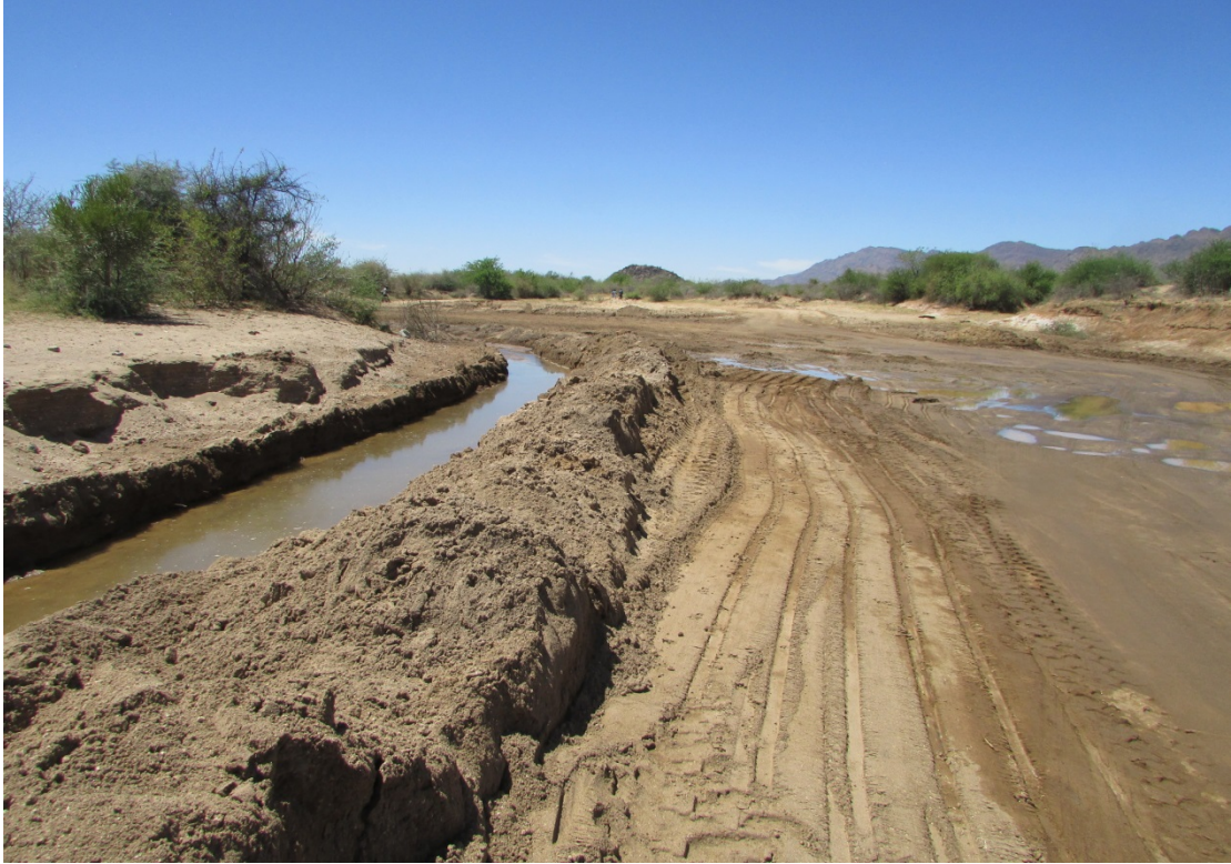
Figure 7: The work being conducted at Point 2.
