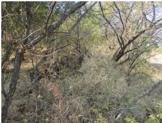
Fig.30: Stone walling on Portion 135.
