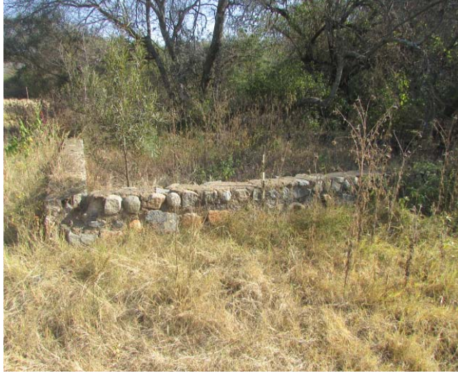
Fig.21: One of the stone and cement structures on the site.
