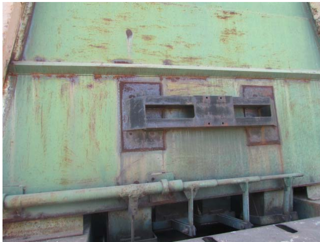
Fig.19: Another view of part of the structure.
