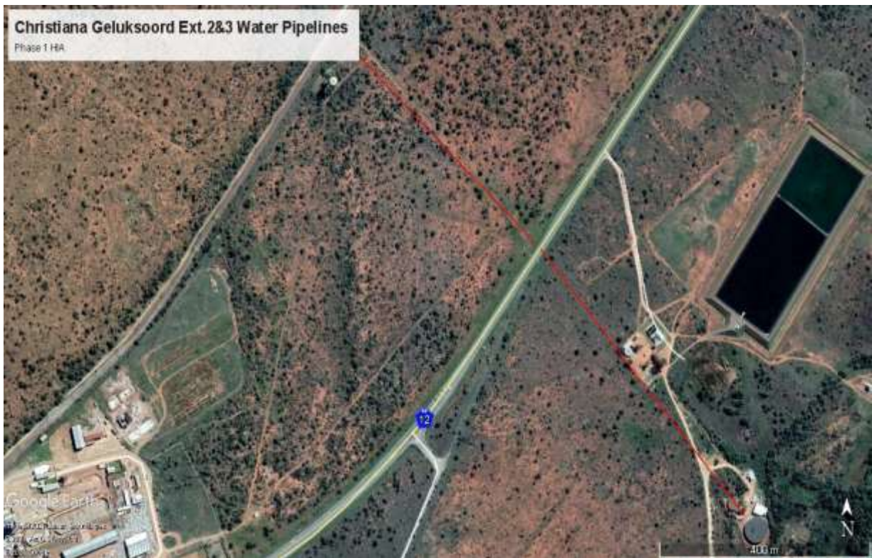
Figure 6: View of a section of the line towards the Christiana water tower and works (Google Earth 2021).
