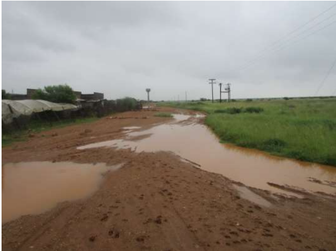
Figure 9: A view of the line towards Utlwanang Water Tower.
