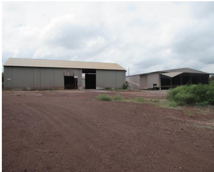
Fig.11: Some of the existing infrastructure at Glenover.
