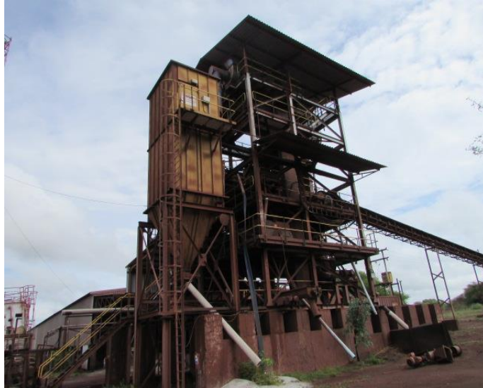
Fig.12: More of the existing mining infrastructure here.
