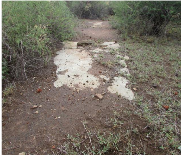
Fig.17: Foundations of another structure on Site 1.
