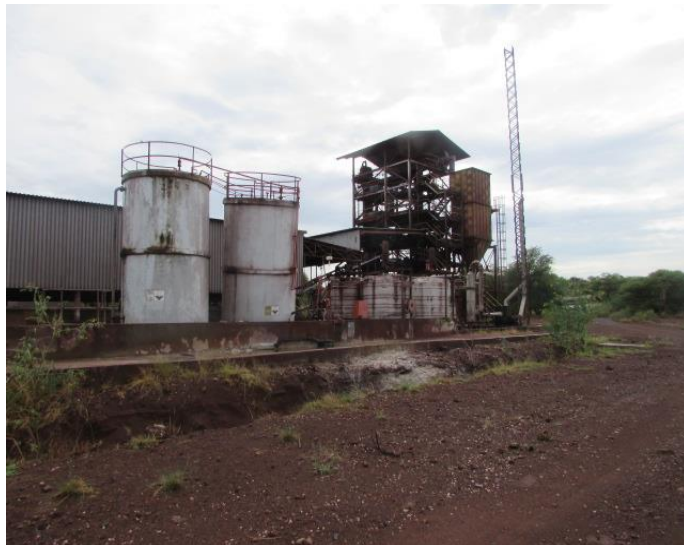
Figure 13: More related structures at the Plant at Glenover. These were erected between 2002/03.
