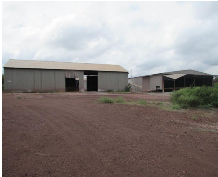
Figure 11: Some of the existing infrastructure at Glenover. These sheds were erected between 2000 & 2010.
