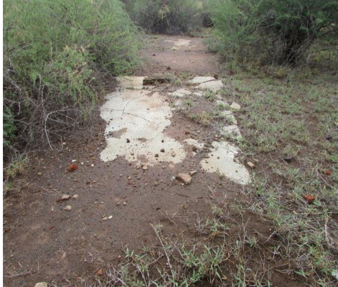
Figure 17: Foundations of another structure on Site 1.
