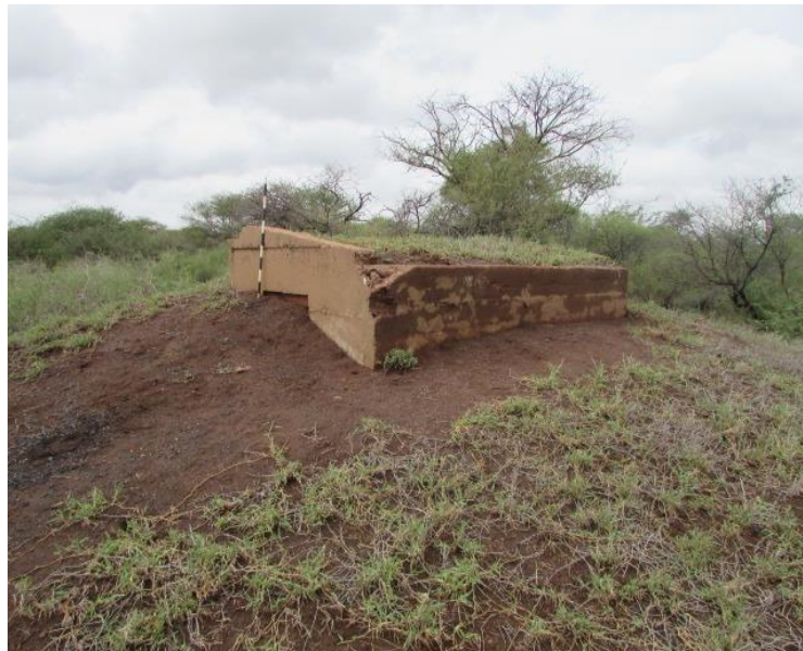
Figure 16: One of the structures on Site 1.
