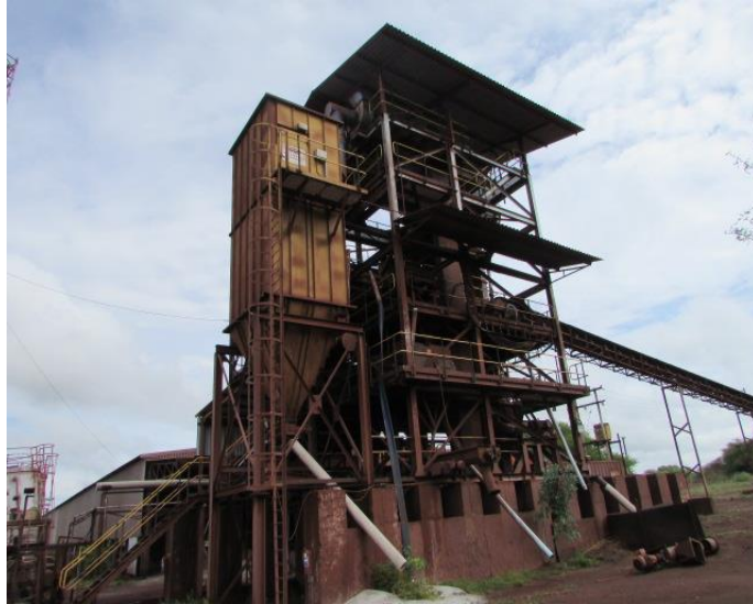
Figure 12: More of the existing mining infrastructure at the Plant area. The Plant was constructed in 2002/03.
