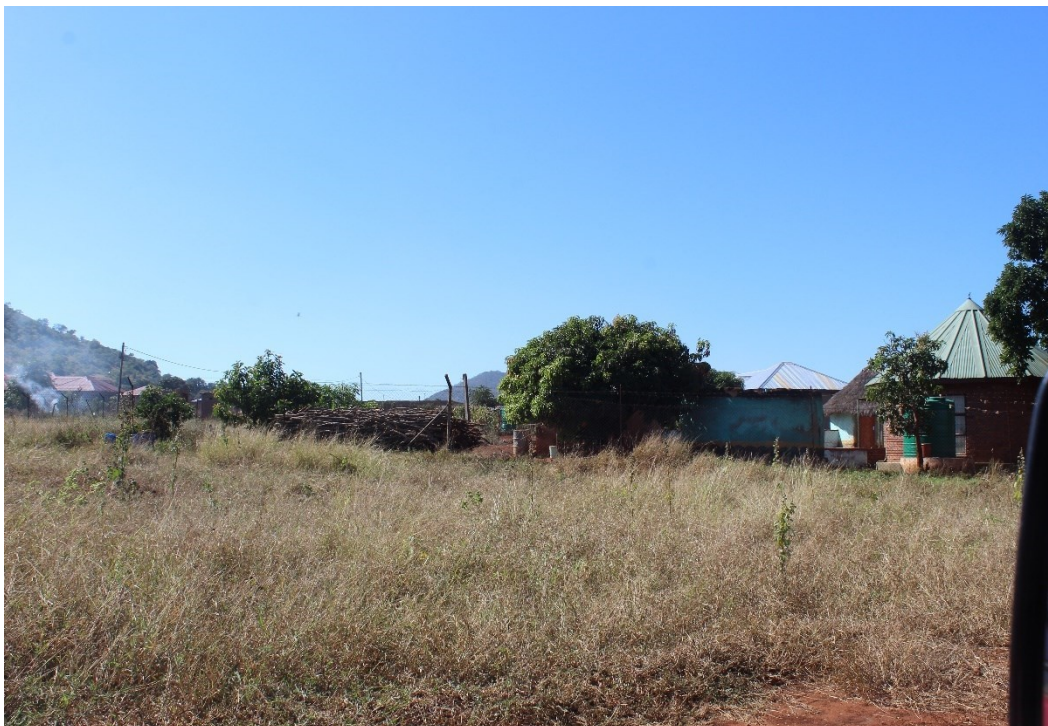
Figure 7: Informal and formal settlement on the eastern boundary of the study area (courtesy Ubique Heritage Consultants).
