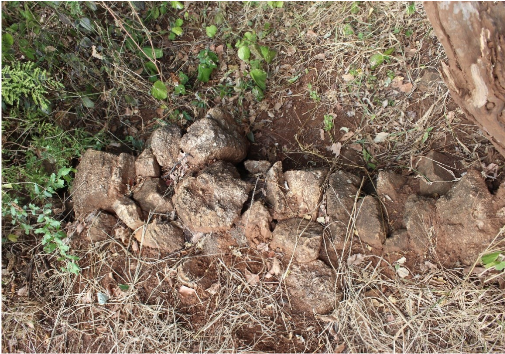
Figure 11: The Site 001 wall feature (courtesy Ubique Heritage Consultants).
