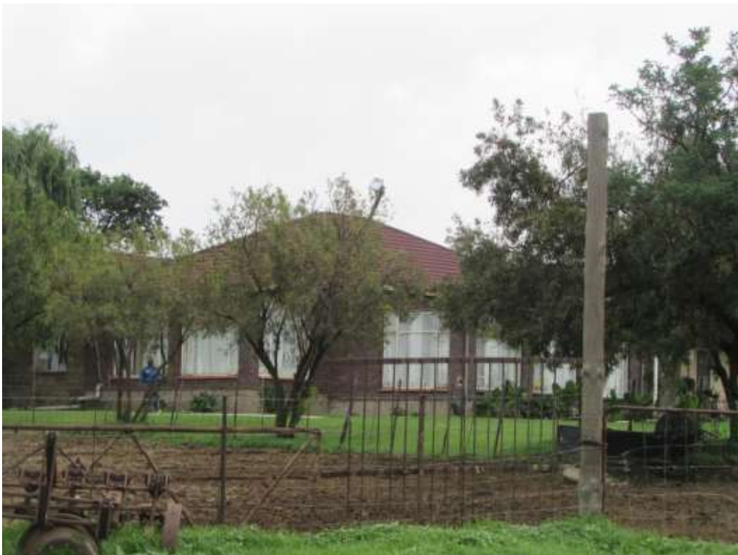
Figure 12: A view of the main house. Sections of the original sandstone is visible.
