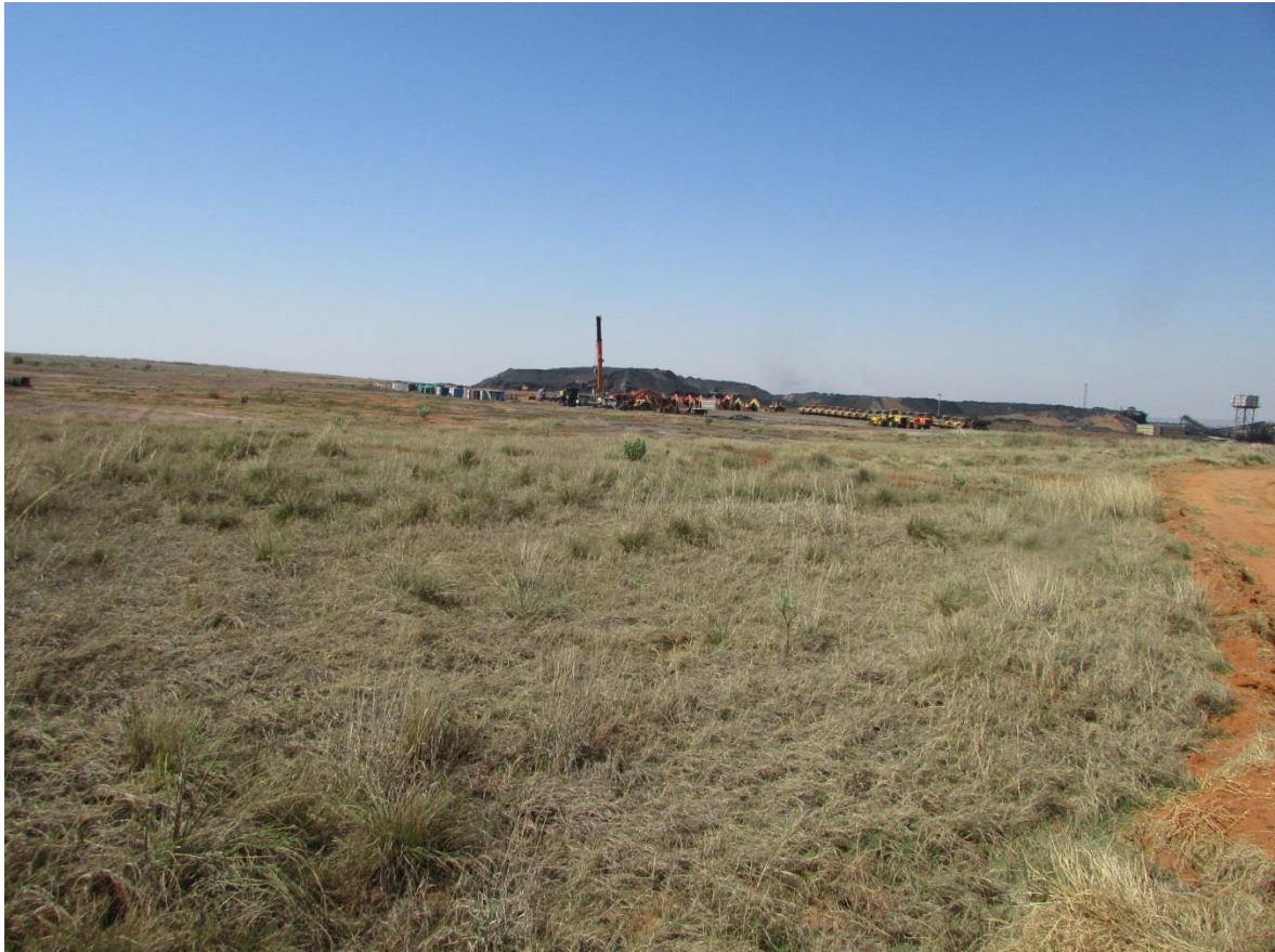
Figure 10: Another section of the Alternative A area. Mining-related activities & developments are evident here.
