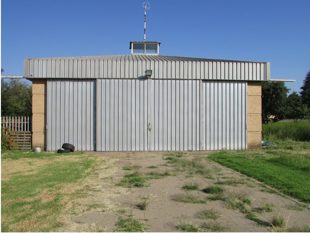
Figure 15: A modern structure (store room) on the property.
