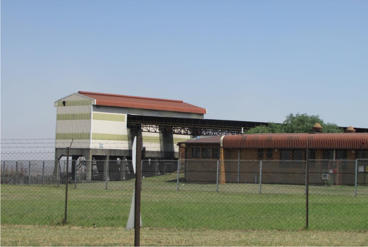
Figure 4: Mining related infrastructure at the Plant area.
