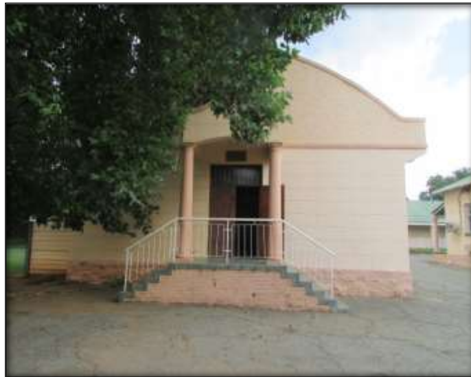
Fig.7: One of the other Salvation Army buildings dating to same time-period. It will also be retained and renovated.
