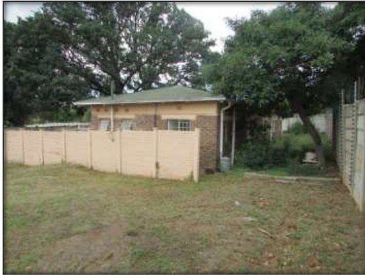
Fig.10: Other recent structures that will be demolished.
