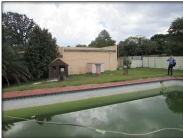
Fig.9: Some recent structures that will be demolished. The swimming pool will also be demolished.
