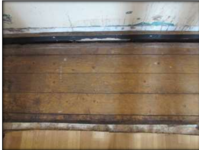
Fig.16: Sections of old wooden floors visible.
