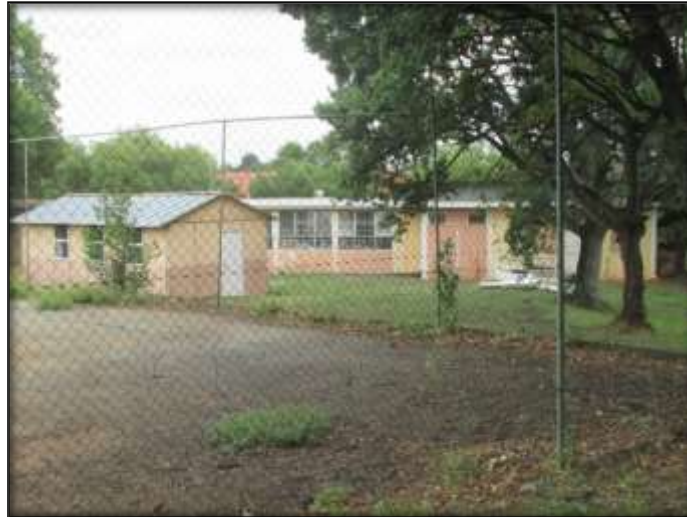
Fig.21: A view of some recent asbestos structures. They will be demolished as part of the development.
