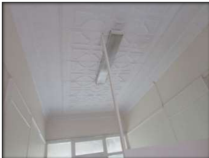
Fig.15: Another section of pressed ceiling.
