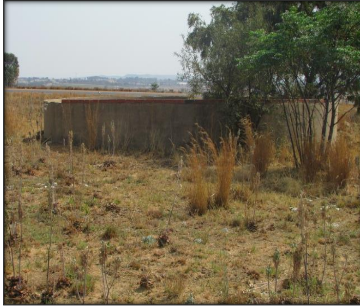
Fig.16: A cement dam close to the grave site.
