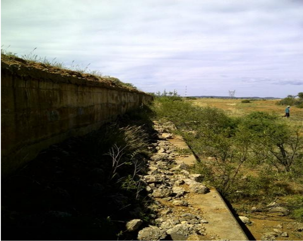
Figure 7: Another view of the site.
