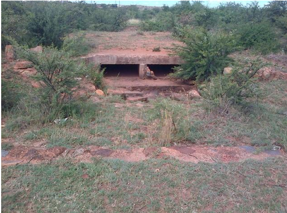
Figure 13: The low-level concrete bridge in the study area.
