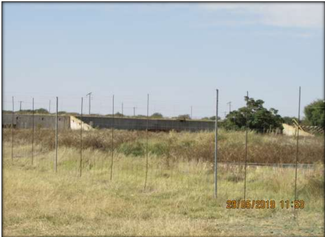
Figure 10: A view of some of the Fertilizer plant structures on the site.
