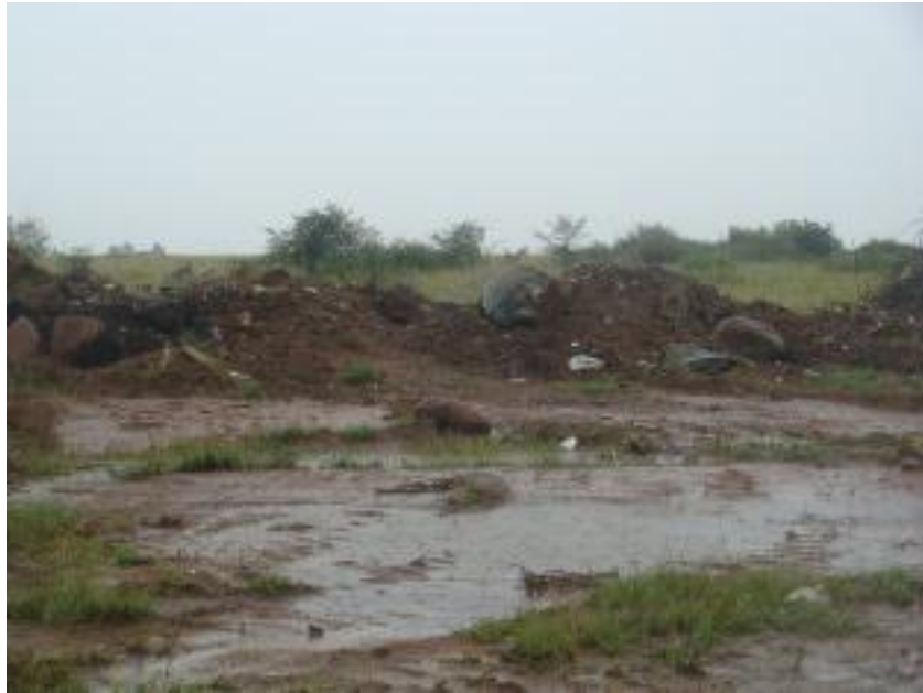
Figure 6: Recent earthworks in a part of the study area.
