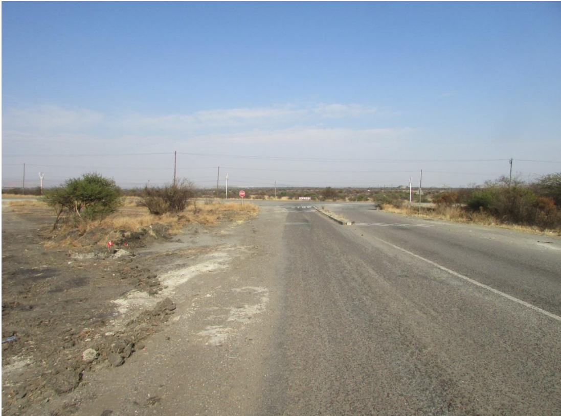
Figure 11: A view down a section of the Option 1&2 route towards the western part of the line.
