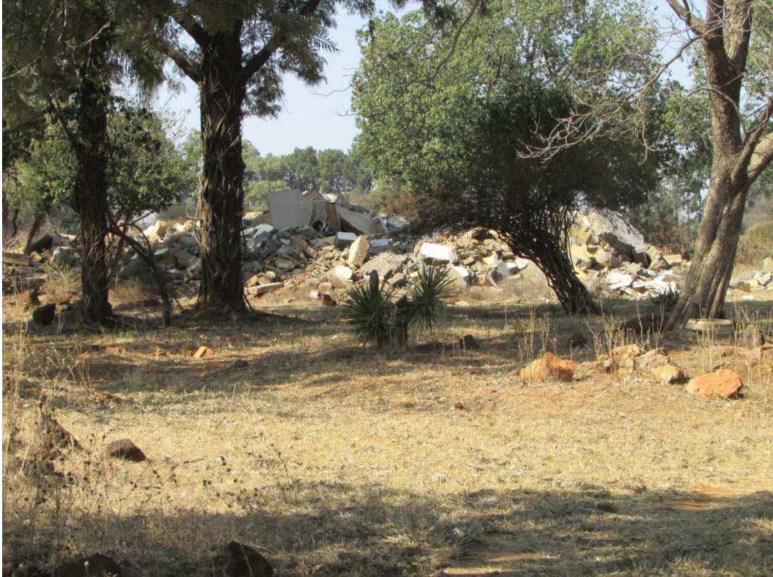
Figure 15: Another demolished homestead on one of the properties earmarked for development.
