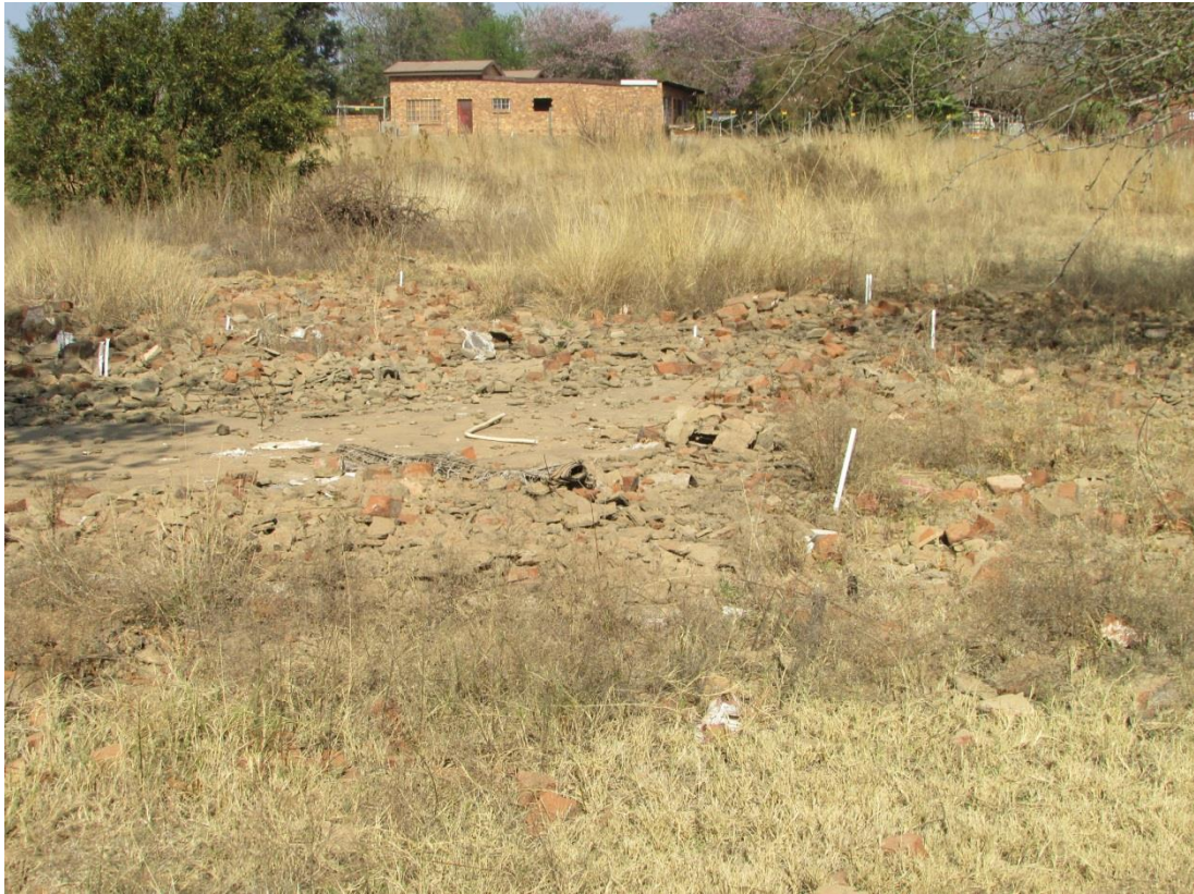
Figure 7: The foundations of a structure on one of the properties. The demolition of many structures is visible throughout the study area.
