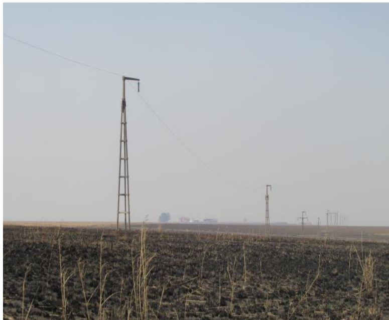
Figure 6: A view showing the old electrical lines running across the site.
