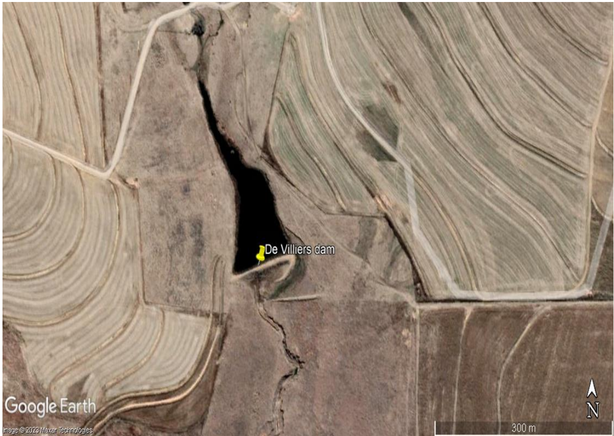
Figure 2: Closer view of the De Villiers Dam area (Google Earth 2023).
