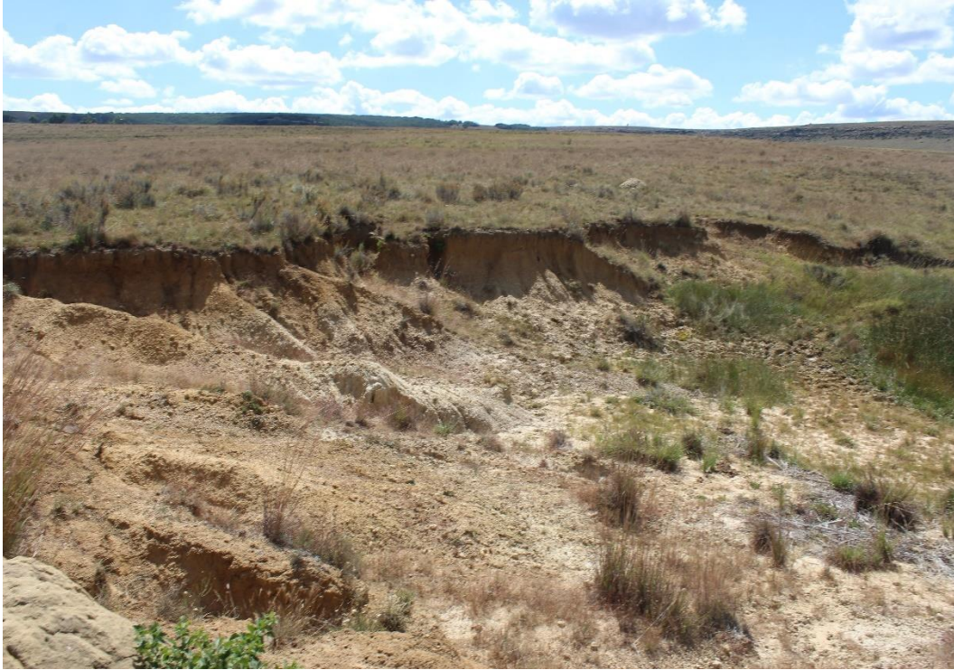
Figure 15: Erosion donga in the Cyprus Dam area.
