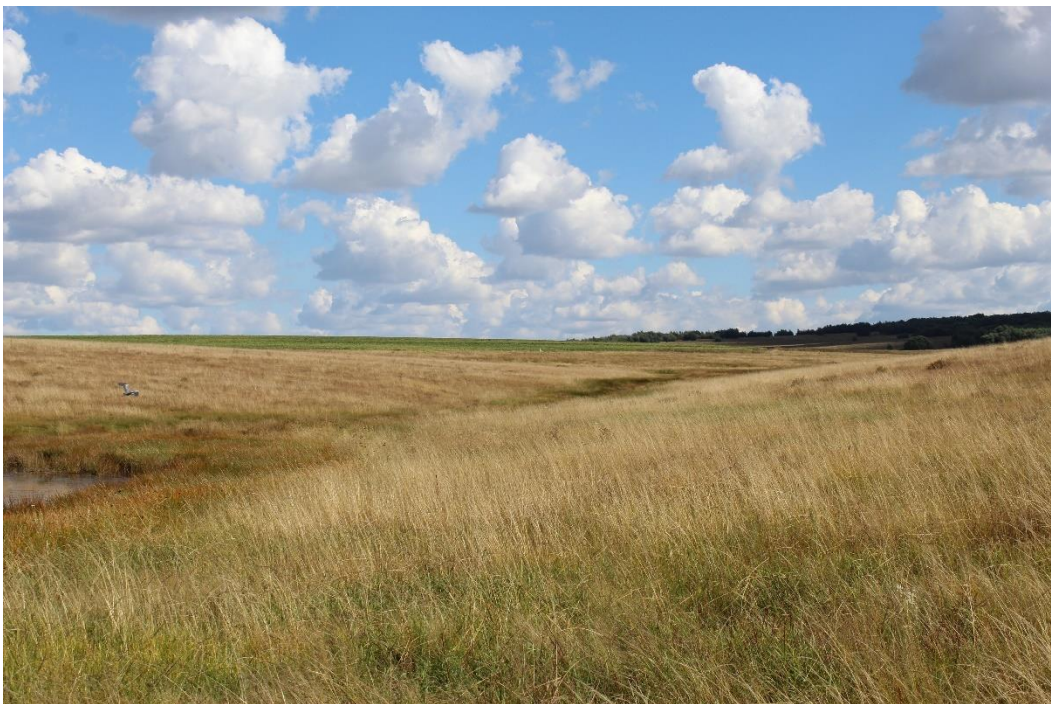
Figure 22: General view around the 3 rd Hills Cottage dam.
