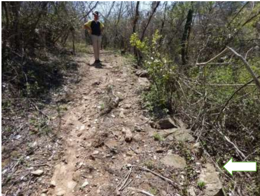
Fig. 15: It is recommended that the existing road be used to gain access to the sites. The road was built up in sections with large stones to support it on the slope.
