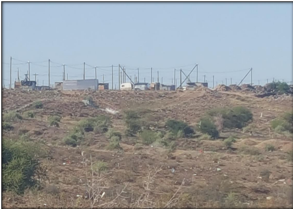
Figure 10: Another view of a section of the study area. Note the established formal and informal housing here.
