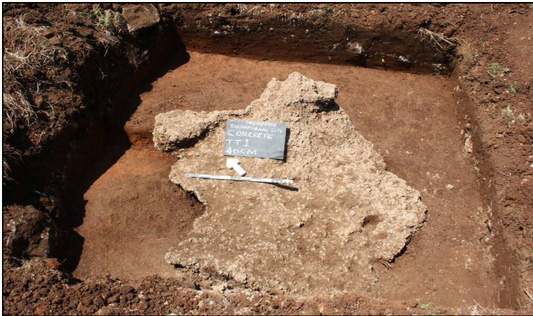
Figure 7: Excavated test trench where concrete rubble was buried by Roshcon contractors.
