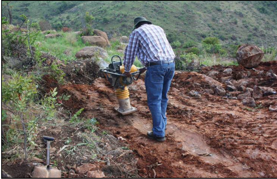
Figure 11: After the removal of concrete slab the open sections were rehabilitated
