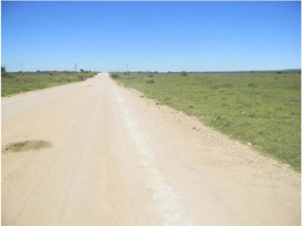
Powerline route along road servitude
