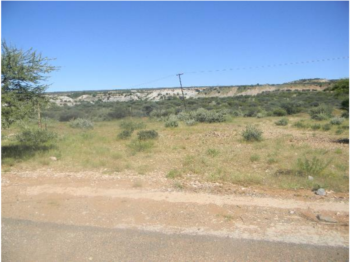
View of existing 22kv powerline running near the site boundary
