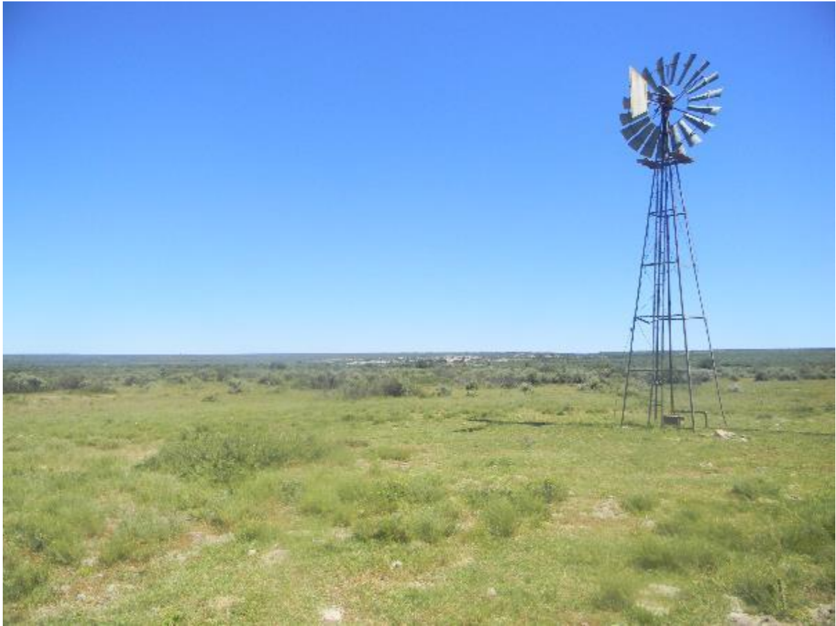
Some of existing infrastructure in the project area
