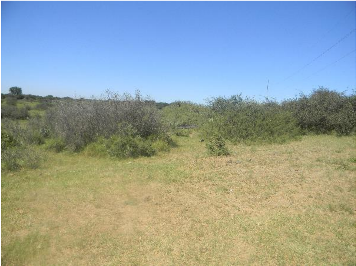
Powerline rout along existing 132kv powerline route
