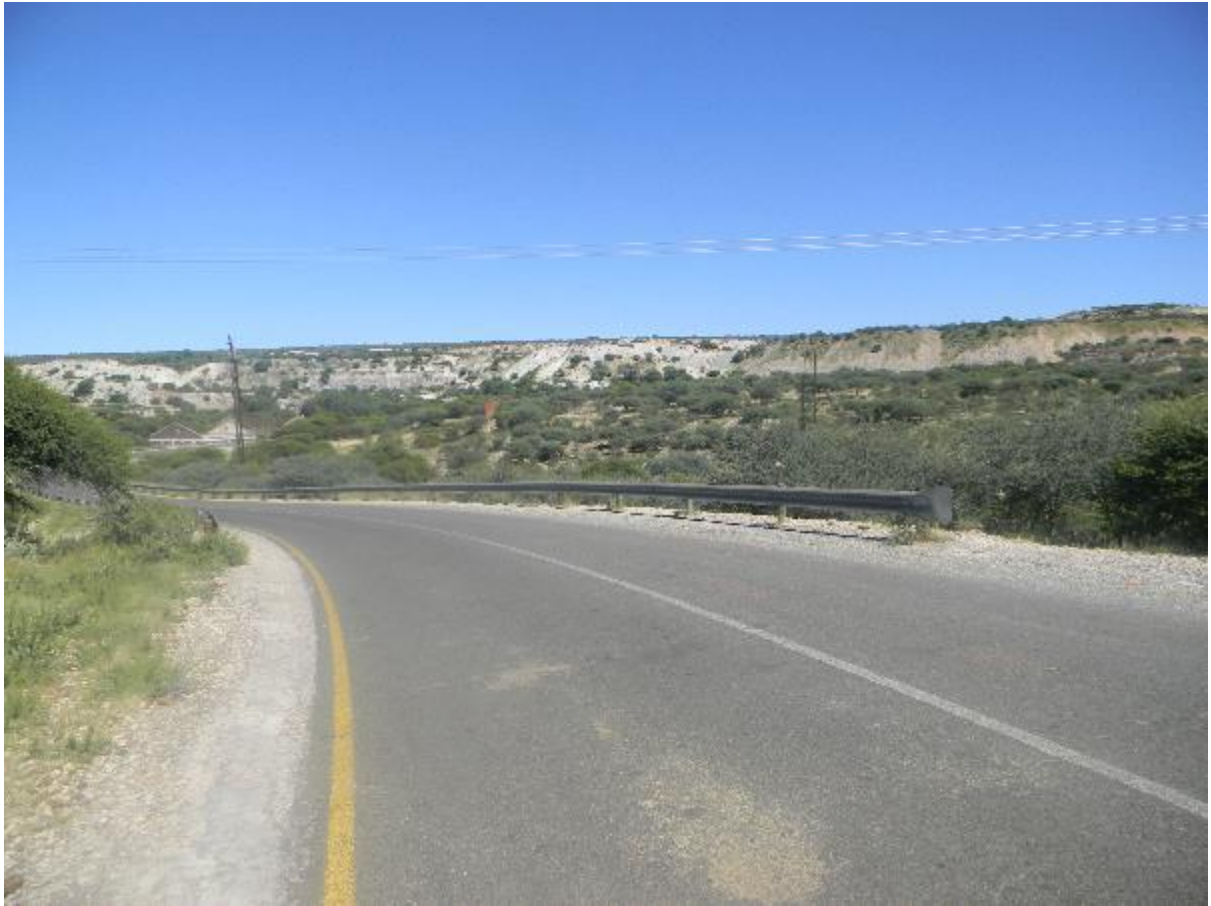
Main road running between site boundary and the substation
