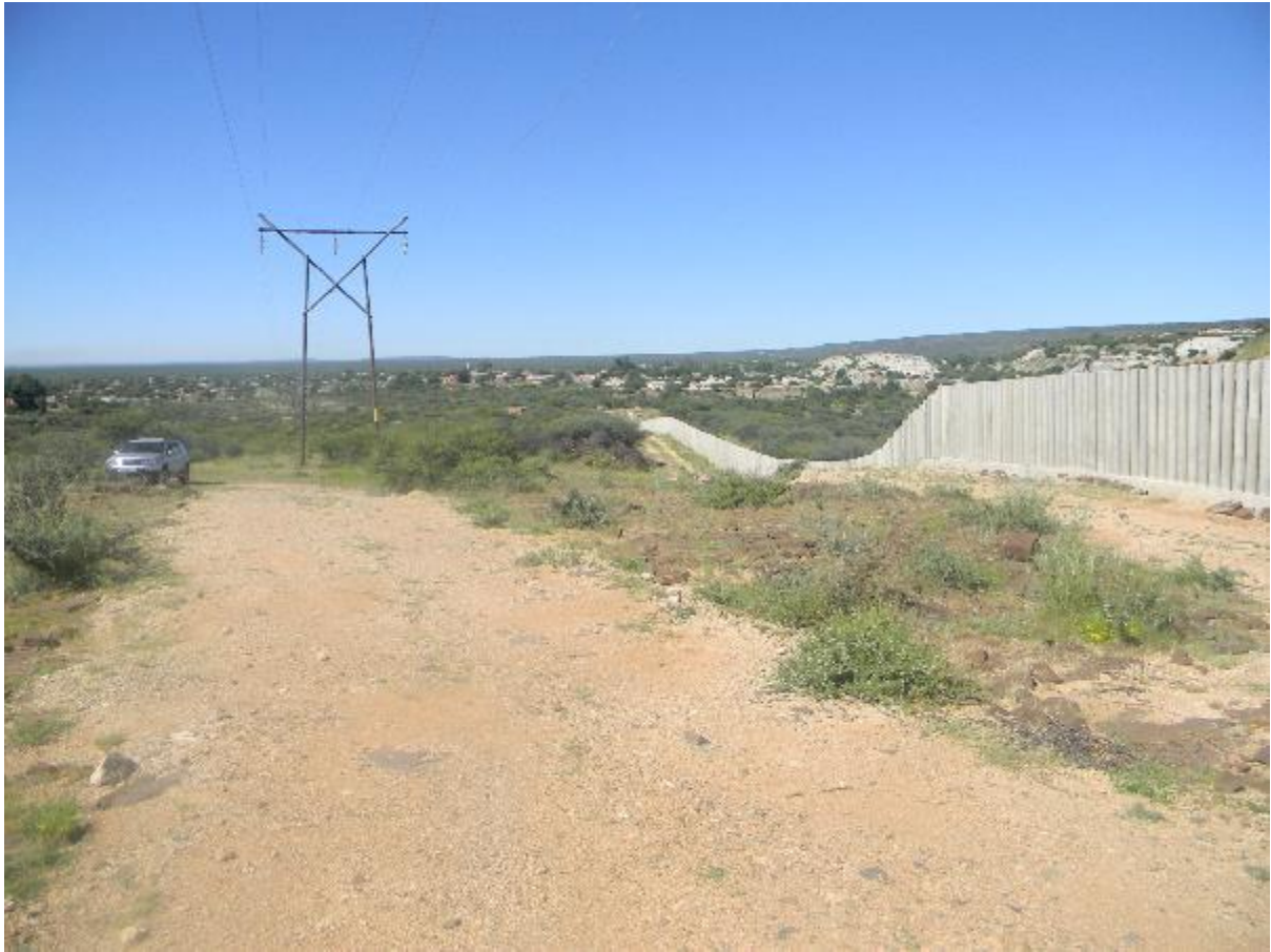
Existing poweline running close to the boundary of the site
