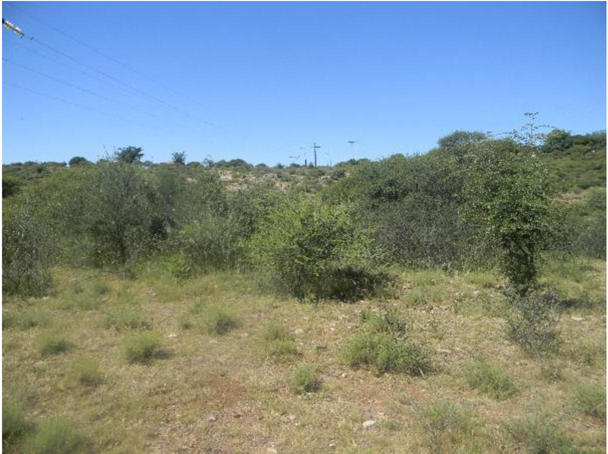
Existing powerline, the proposed powerline will run parallel to the existing line on the right
