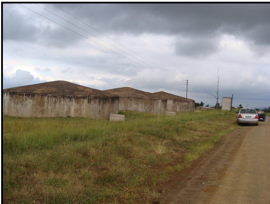
Figure 55: Existing dams that will be upgraded and improved as a result of this project (GPS co-ordinates S 27° 57' 14.95" E 31° 46' 22.83")
