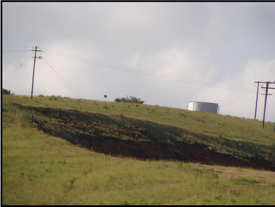
Figure 52: Site of existing reservoir which will be upgraded and improved as a result of this project (GPS co-ordinates S 27° 56' 26.99" E 31° 49' 38.08")
