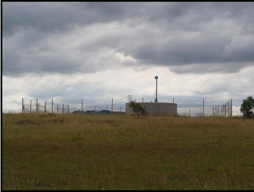
Figure 36: Small reservoir on hill which will be improved and upgraded during this project (GPS co-ordinates S 27° 51' 13.9" E 31° 42' 16.0")
