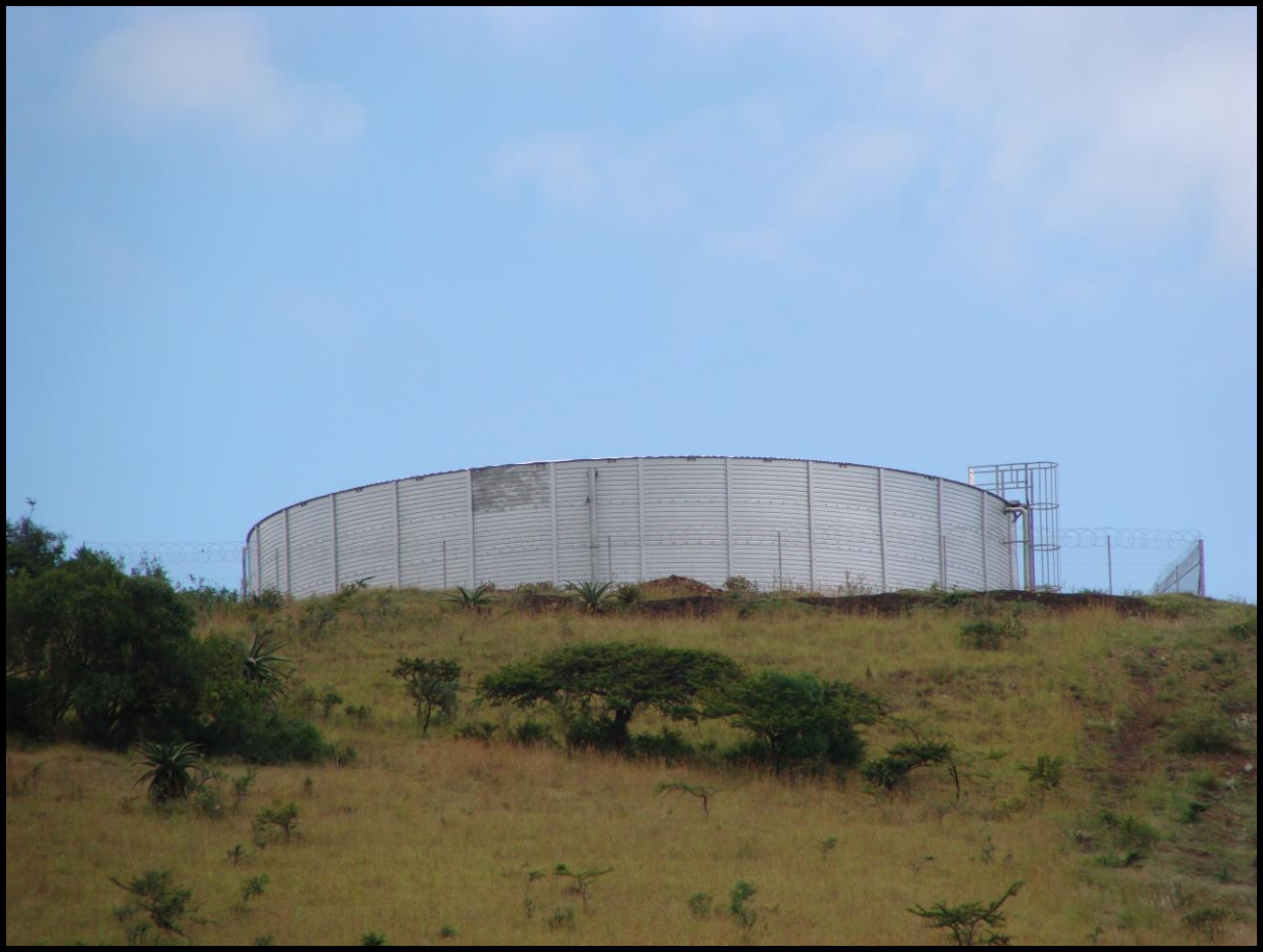
Figure 27: Reservoir on top of hill which will be improved and upgraded as part of the pipeline project (GPS co-ordinates 27° 51' 34.93" E 31° 47' 15.43")
