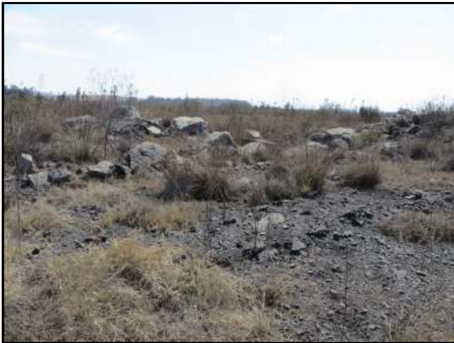
Figure 15: View of the unconsolidated, chaotically oriented polymict boulders of Karoo lithologies that indicate that the PCD area has been subject to landfill and rehabilitation (Waypoint KK9; see Figure 4).
