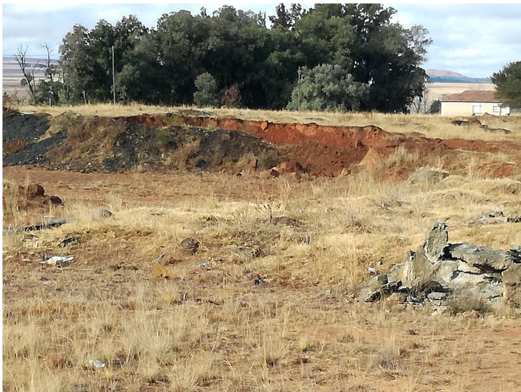
Figure 15: Highly oxidised soils in the cut profile (and infill of building refuse).
