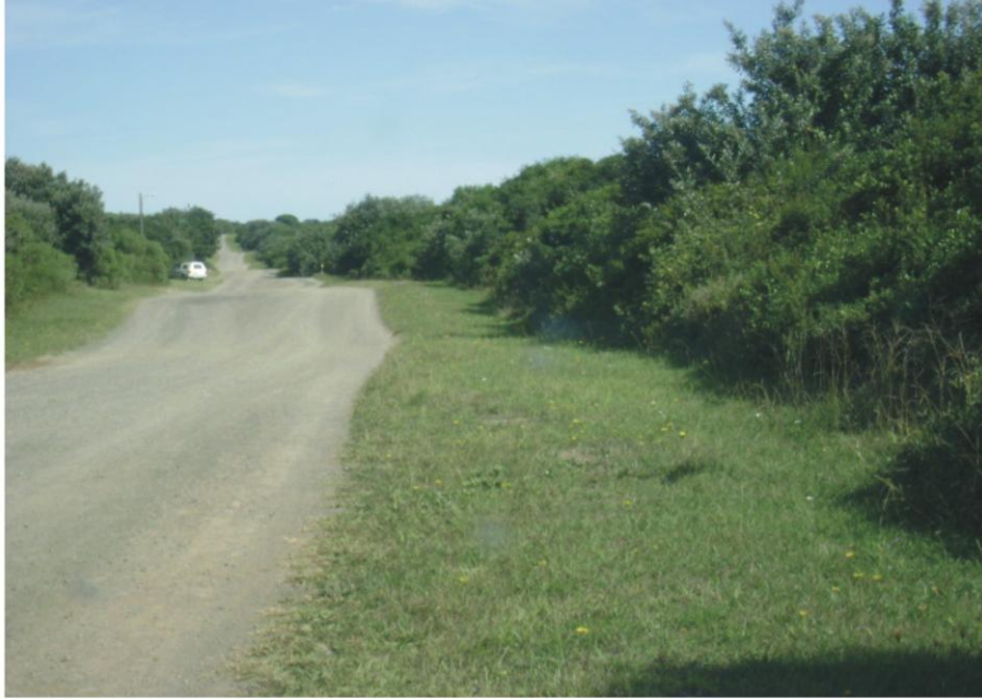
Figure 9. Pipeline section east of the BWRO, located on Nanaga Frm sediments.
