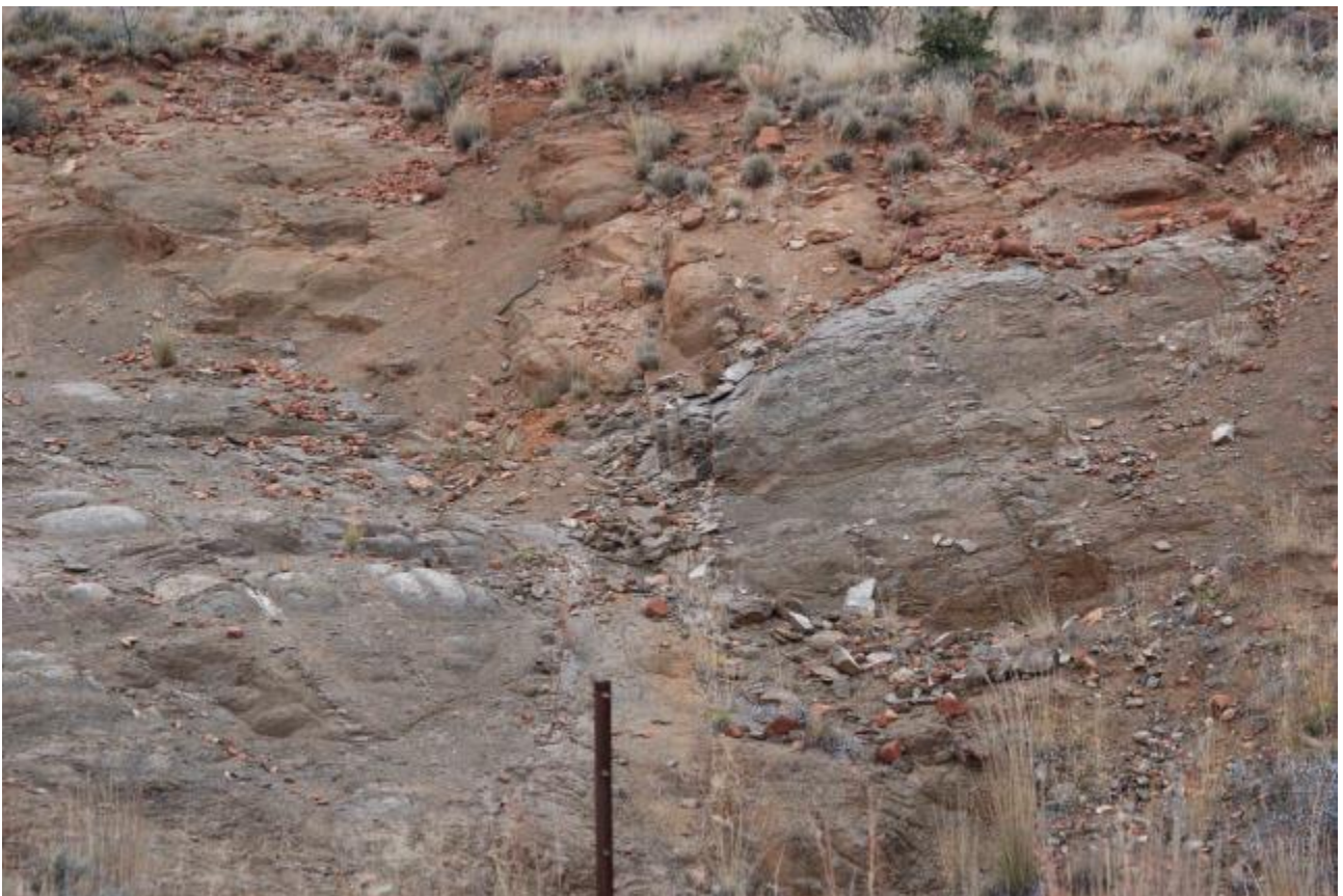
Figure 7: Bontehoek borrow pit: top : proposed site of new borrow pit showing calcretised rotten dolerite exposed by a test pit; bottom : dolerite exposed in old borrow pit adjacent to new site.
