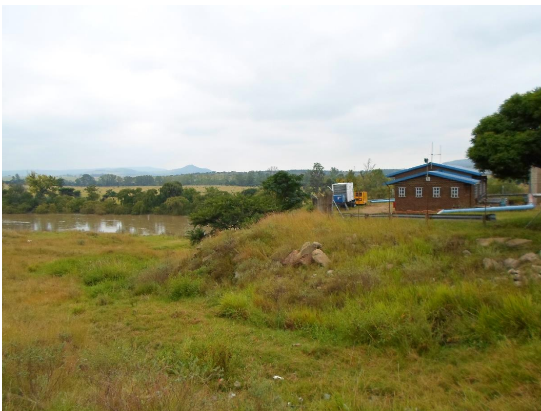
Figure 8: Western section showing the pump house built on artificially raised ground (Photo by JvdW).
