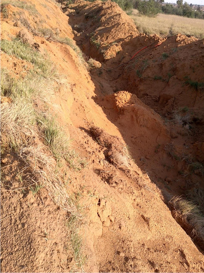
Figure 13: Stop 6 showing another trench and deep sand.
