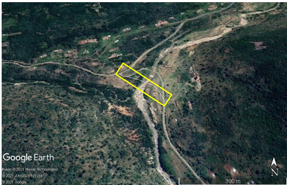
Figure 1: Google Earth map of the proposed causeway on L3097 across the Mdumbeni River with the section (white line) shown within the yellow outline. Map supplied by EnviroPro.
