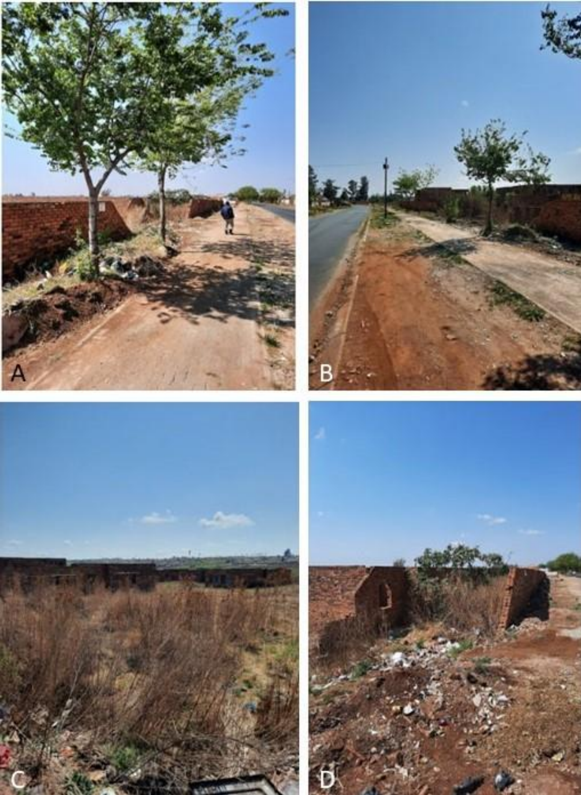
Figure 5: Protea Glen Ext 1 Site photographs. A-B – views north and south along the western border to the site. C-D – views alongside the partially built structures showing disturbance and dumped rubbish. No dolomite and no fossils seen.
