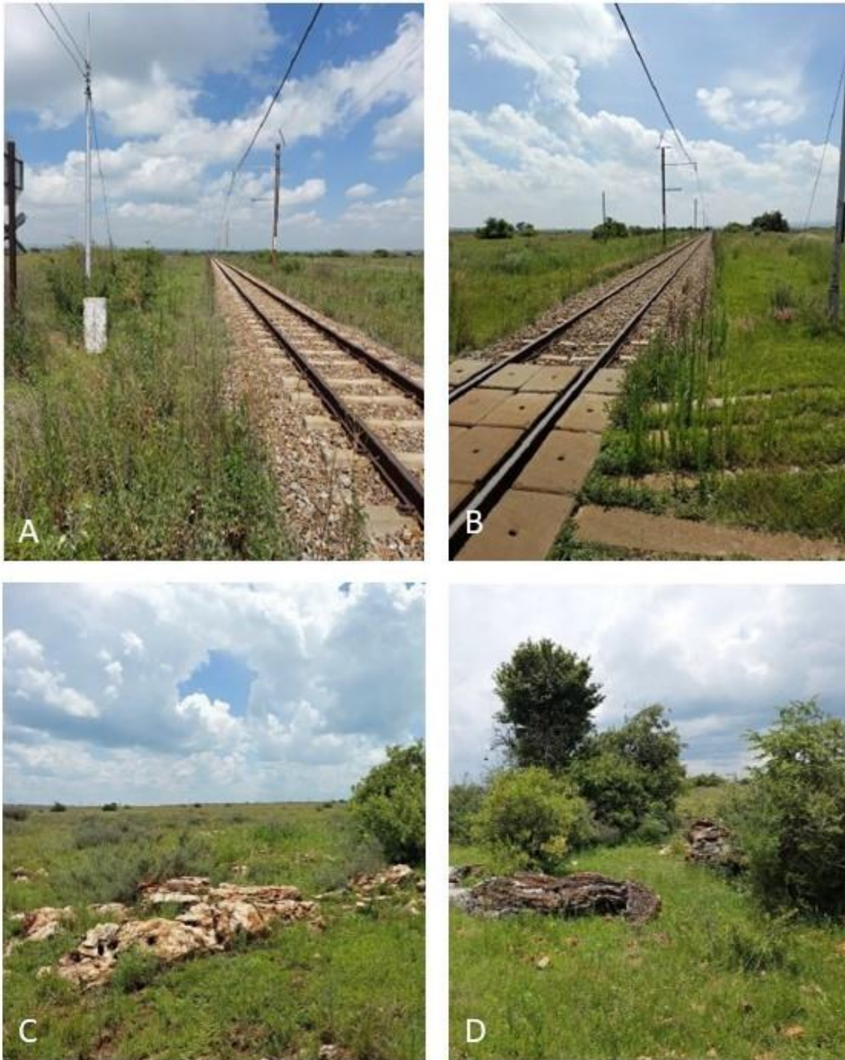
Figure 6: Site visit photographs for Mopane Solar PV 3. A-B – the railway transecting the farm. C – outcrop of chert in the foreground. D – outcrop of dolomite but no stromatolites present.
