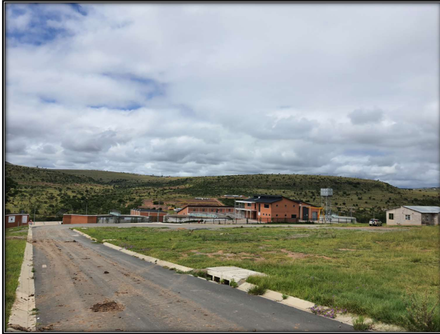
Figure 7: Existing Water Treatment Works (central view)
