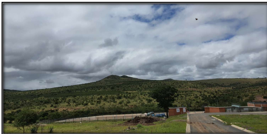
Figure 8: Existing Water Treatment Works (southern view).
