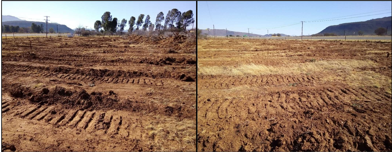
Figure 14: Vegetation clearance next to the R61 indicates the absence of outcrops
