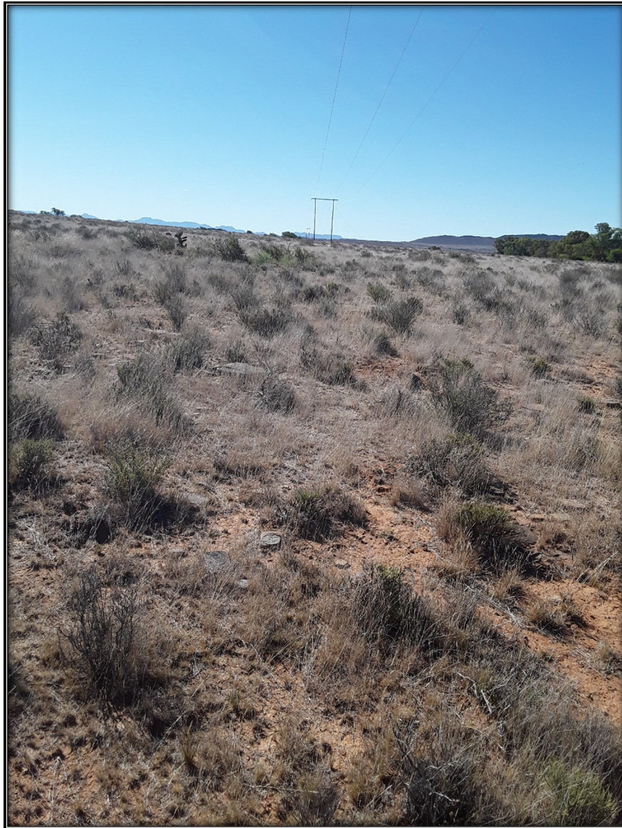
Figure 10: Proposed powerline right next to the existing powerline. Grassy vegetation with isolated sandy patches. No fossiliferous outcrops were identified.
