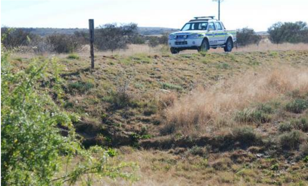
Figure 12. Site of the proposed agricultural underpass showing road bed raised on alluvial surface.
