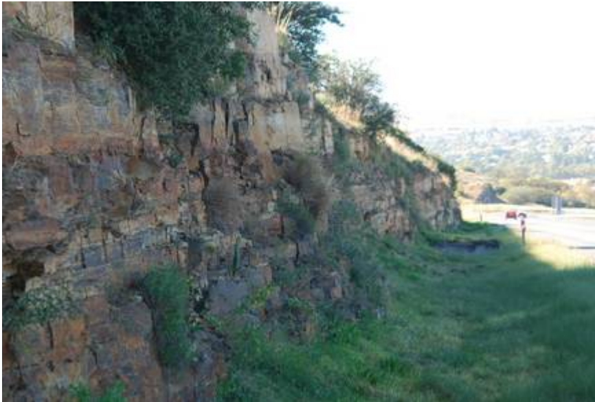
Figure 5. Southern end of the climbing lane cutting showing coarse siltstones and sandstones. The small roadcutting in the middle distance is that composed of dolerite north of the correctional services intersection.
