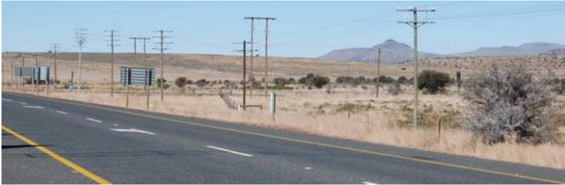
Figure 10. Intersection between N10 and R61 – built up on alluvial plain.
