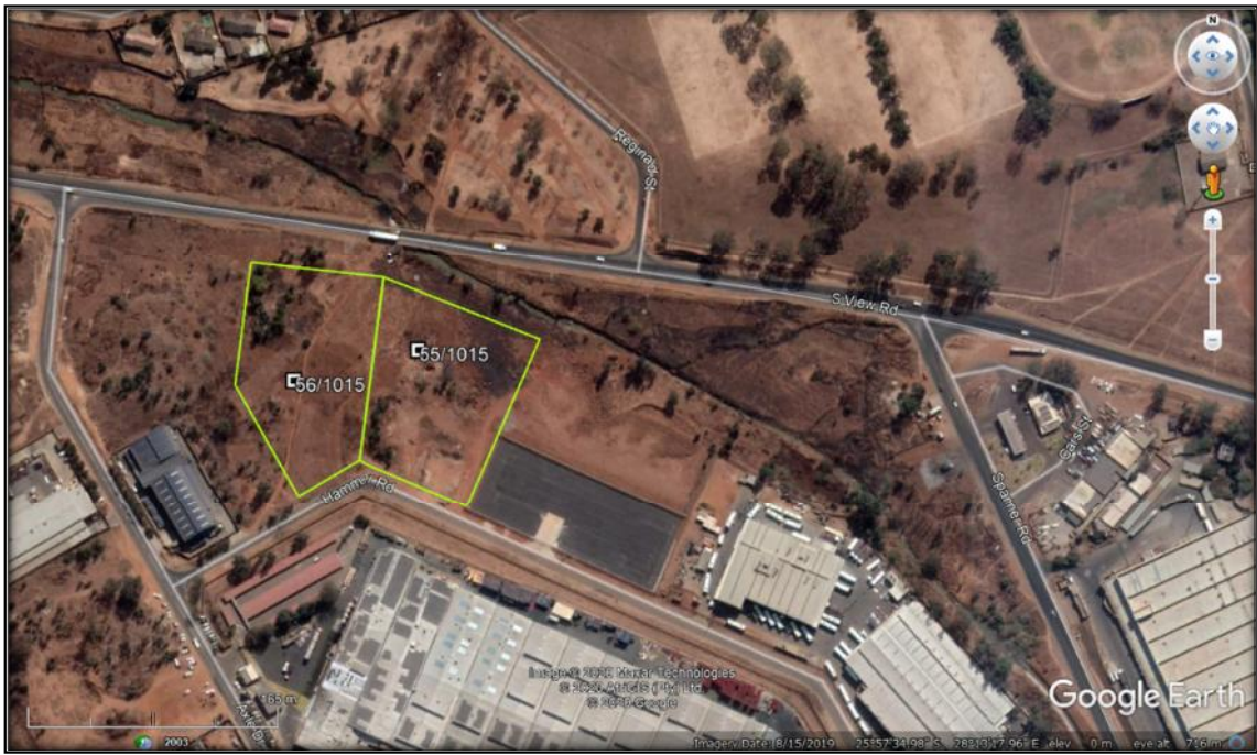
Figure 2: Close-up Google Earth Image (2020) indicating the locality of the proposed Clayville Truck Yard ablution blocks and wash bay situated on Portion 55 and 56 of Erf 1015, Clayville X11, Ekurhuleni Metropolitan Municipality, Gauteng Province. The proposed development is indicated in green.
