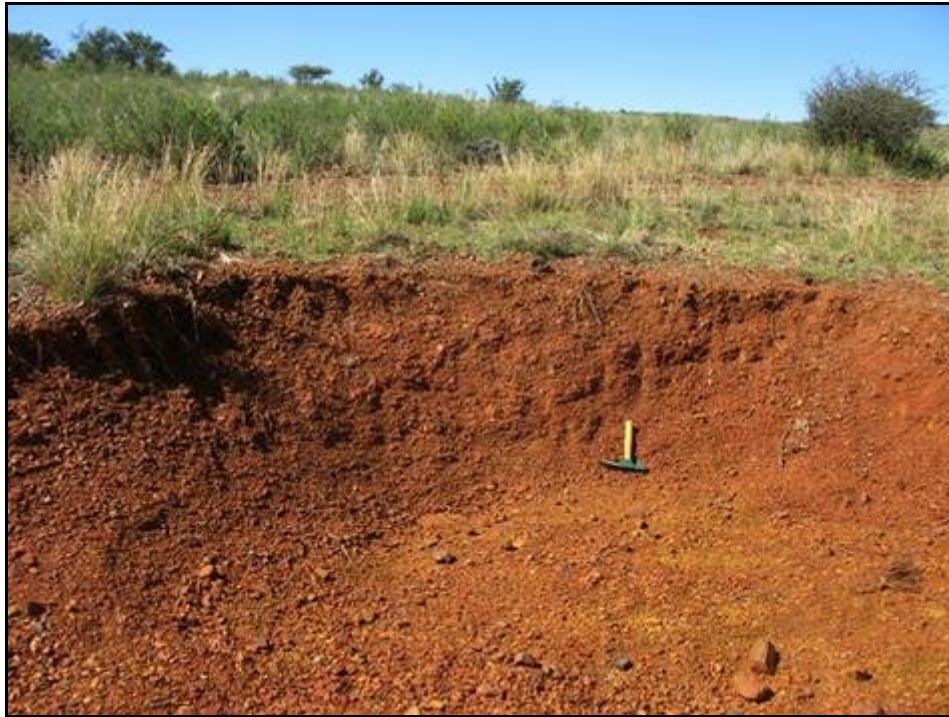
Fig. 16. Borrow pit into thick surface gravels and underlying weathered BIF, north of Metsimetala Village (Loc. 503) (Hammer = 27 cm).
