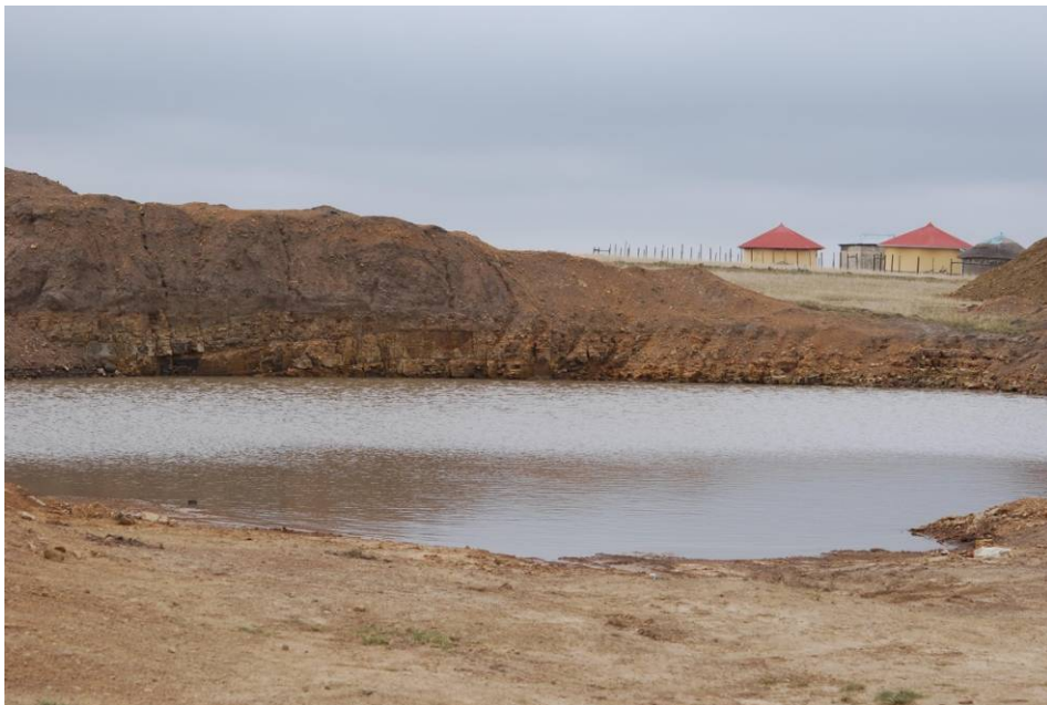
Figure 4. Borrow pit 344 BP04 largely flooded with rain water.
