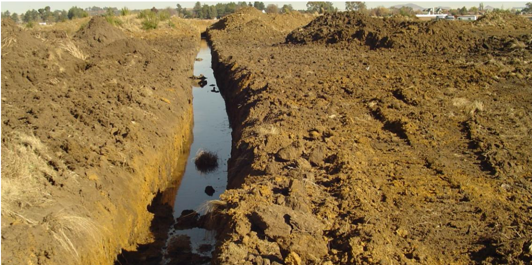
Figure 3: Trench showing the thickness of soil cover
