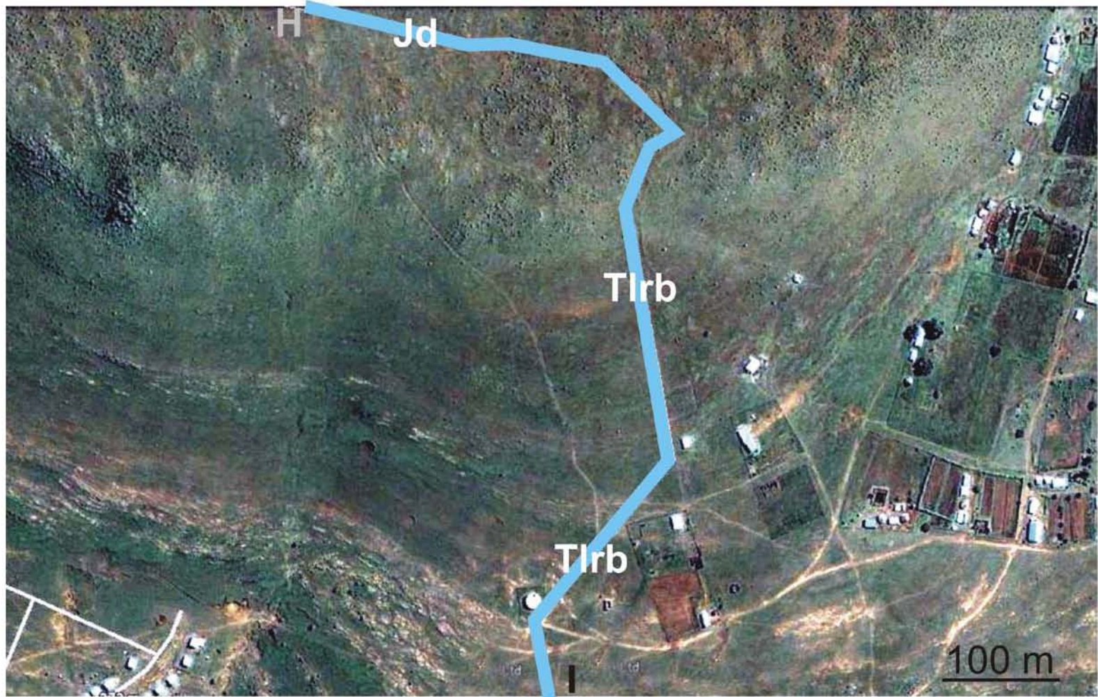
Figure 17. Pumping Main. Aerial view of Section H - I. Burgersdorp Formation sandstones and mudrock ( Tlrb ) are exposed along the foot of the mountain to the northeast of Tsomo town.
