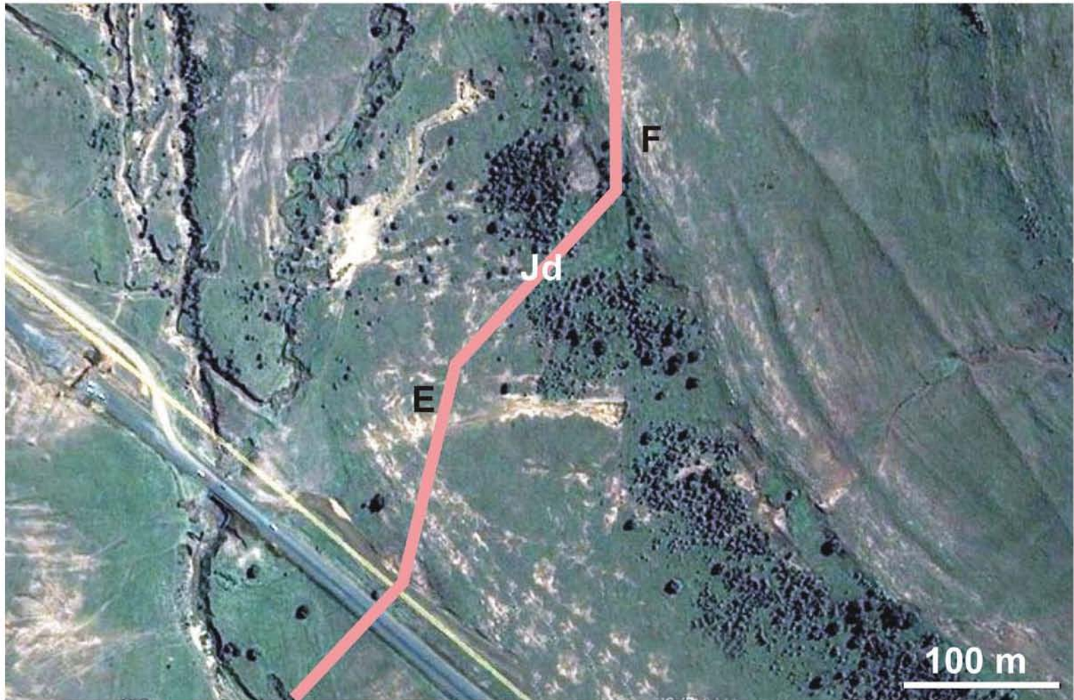
Figure 14. Gravity Main. Aerial view of Section E - F. The section is underlain by a dolerite dyke. Colluvium make up the superficial component.
