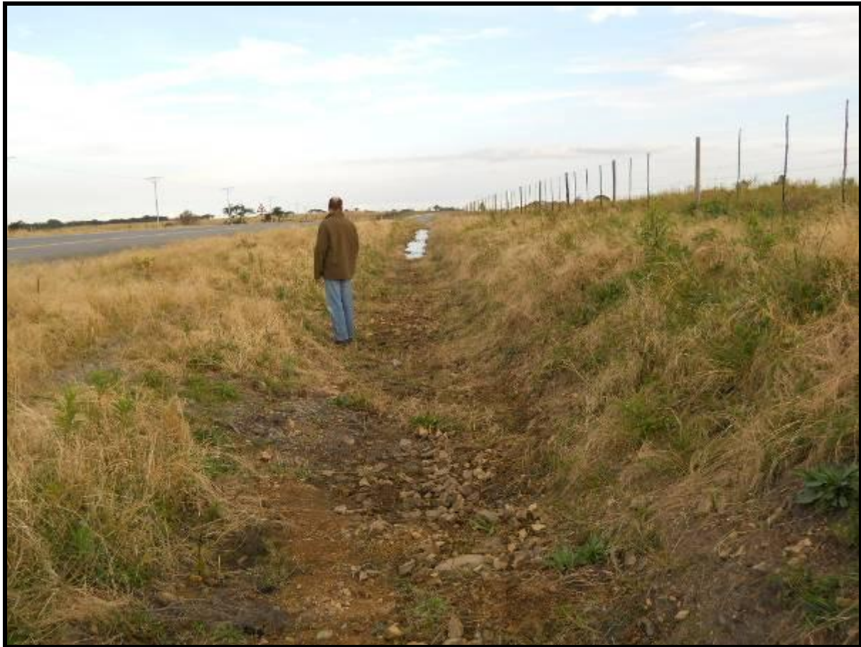
Figure 6.3 Outcrop of Balfour Mudstone in Road Cutting (S32.56900; E27.95011)
