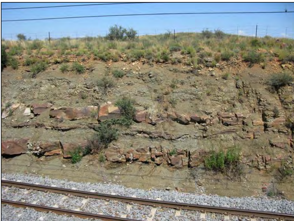
Fig. 6. Good vertical sections through Adelaide Subgroup sediments along railway cuttings. Lenticular channel sandstones (secondarily coated with rust) are interbedded with grey-green overbank mudrocks.
