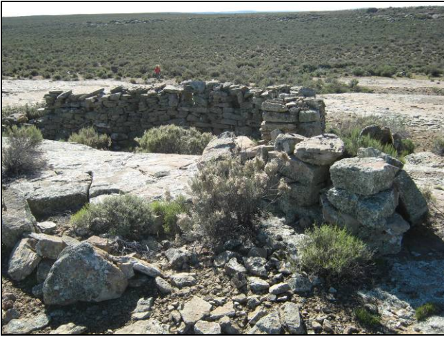
Figure 51: Well preserved stone walling with gun ports alongside a bedrock outcrop at JKV73.
