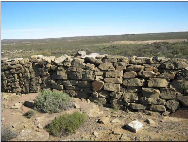
Figure 44: The stone boundary wall at JKV77, a very well preserved section.
