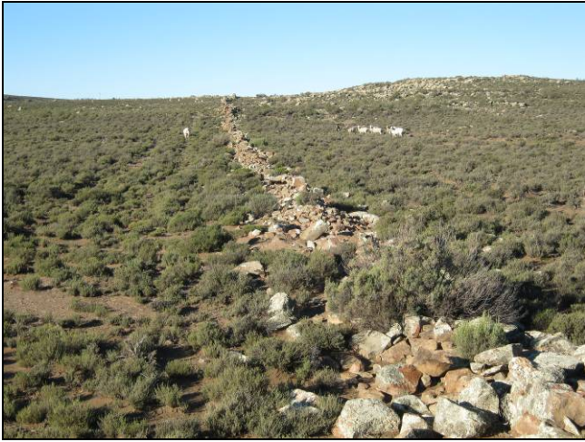
Figure 42: The stone boundary wall at JKV20 showing poor preservation.
