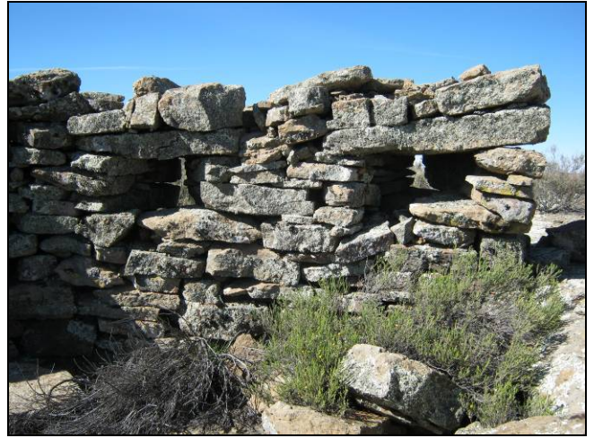
Figure 52: The fully preserved gun ports at JKV73.
