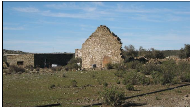
Figure 72: Ruin and outbuilding.
